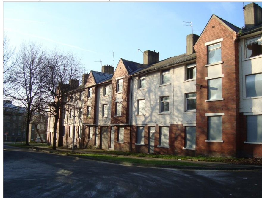
Figure 6: Former tenement block featured red brick and white PVC windows (taken 16/01/2012)
