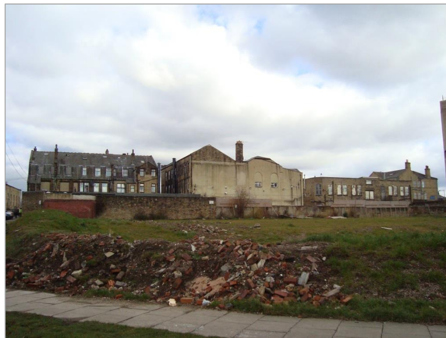
Figure 5: Unattractive rear elevations of buildings fronting Westgate (taken 13/03/2013)
