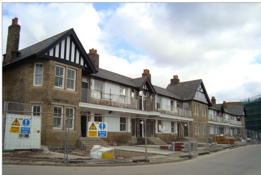
Figure 4: Refurbishment of buildings underway (taken 13/03/2013)
